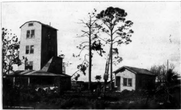
Left—This frame house of E. W. Crane, Hallendale, sheltered 10 neighbors, 110 chickens, three dogs and a cat during the storm and came through without damage. It is sixteen feet square at the base and fourteen feet square at the fourth floor. Mr. Crane lived formerly in North Dakota and built his house to stand. Right—The Alhambra, a small boarding house in Miami. The only damage was caused by water. The wood shingle roof is in perfect condition although laid fifteen years ago. Seven boats and barges were driven into the yard by wind and waves.
